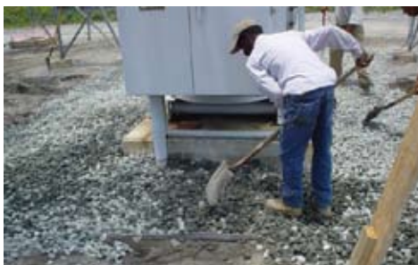
Stone is smoothed to grade level.
