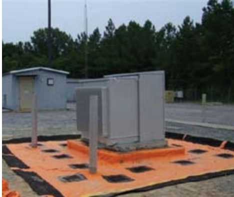
Laying out of blanket sections.
