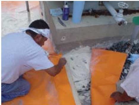
Fitting and gluing sections together.
