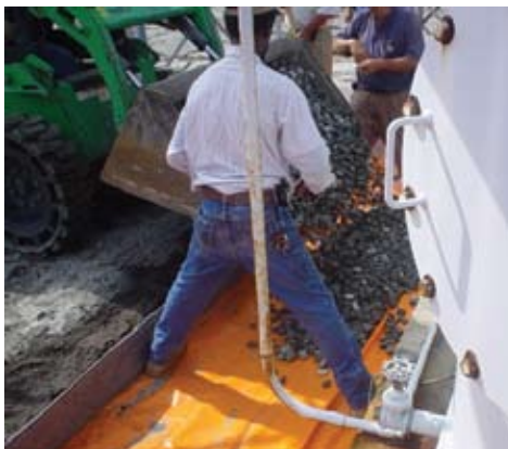
Side wall held in position while stone is applied.
